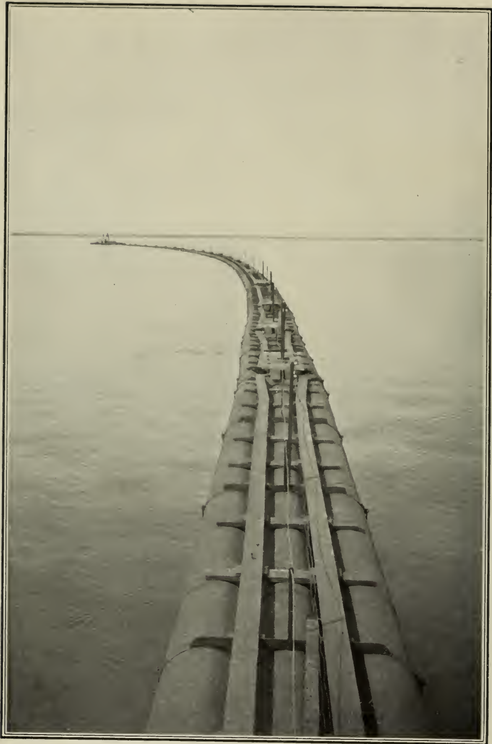
FIG. 27. PIPE LINE OF HYDRAULIC DREDGE J. ISRAEL TARTE.
